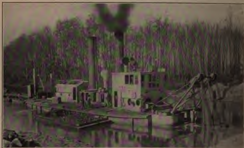
Hydraulic Dredge Operating on New York State Barge Canal. Figure 108.
